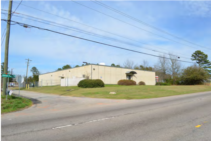
Adjacent AT&T building.
