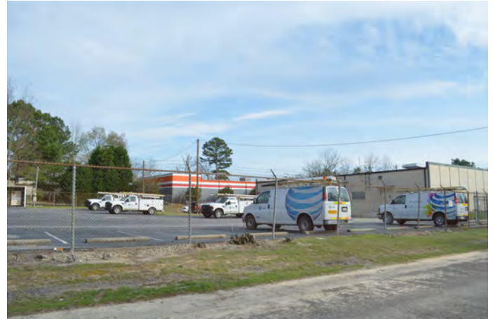
Adjacent AT&T building.
